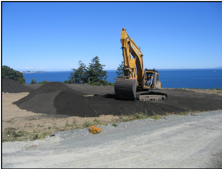
Photograph 2: Fabricated soil containing biosolids, land clearing residuals and fill sand applied at a mine site near Victoria, BC.
