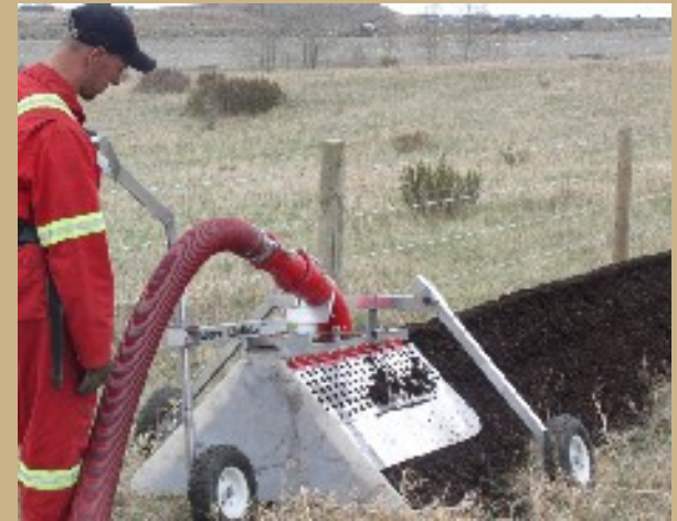
Country Hills Feeder Main, Calgary EcoBerm installation
