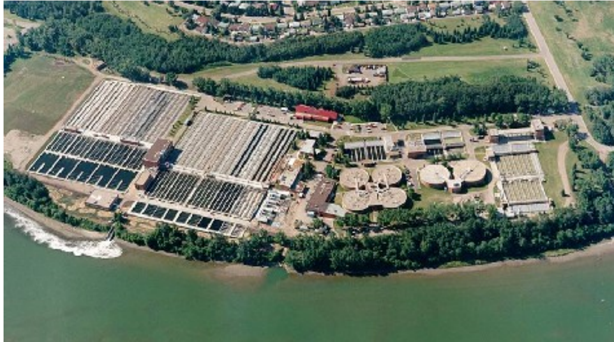
Gold Bar WWTP
